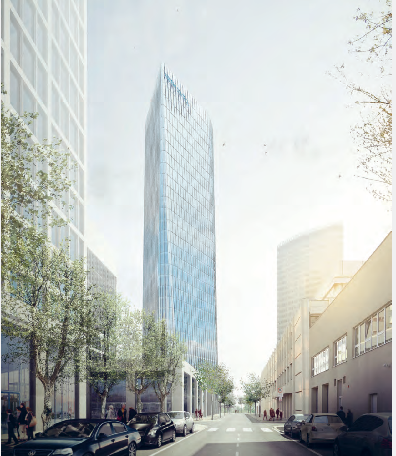
Austro Control Tower. AZPML (Alejandro Zaera-Polo y Mainer Llaguno Architecture). Schnirchgasse 11, Viena, 2015.
