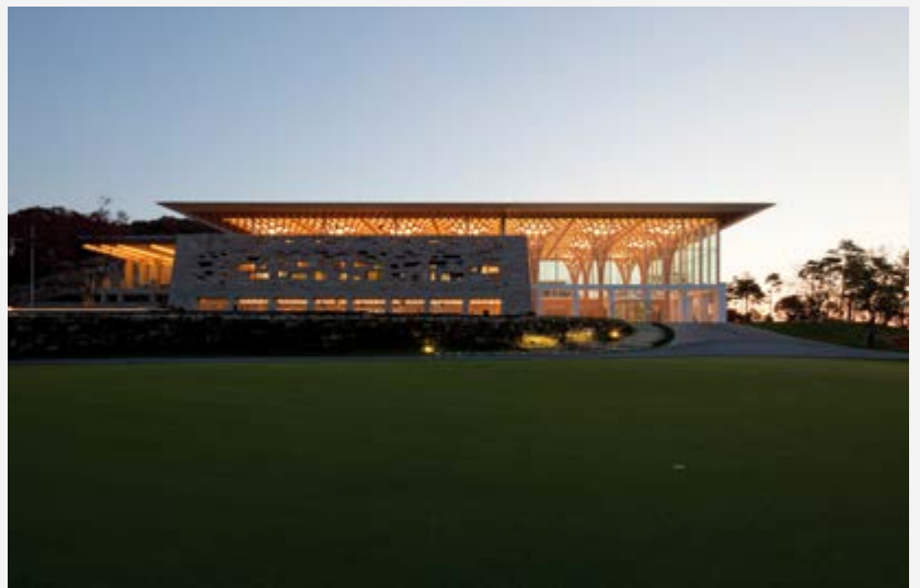
Haesley Nine Bridges Golf Club House (Kyeong Sik Yoon / KACI + Shigeru Ban Architects, Yeosu, Corea del Sur, 2009). Fotografía: Hiroyuki Hirai. Haesley Nine Bridges Golf Club House (Kyeong Sik Yoon / KACI + Shigeru Ban Architects, Yeosu, South Korea, 2009). Fotografía: Hiroyuki Hirai.
