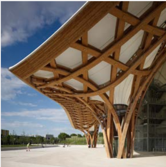
Centro Pompidou en Metz (Shigeru Ban Architects, Metz, 2010). Techo de madera laminada en un patrón entrelazado hexagonal. Fotografía: Didier Boy de la Tour. Centre Pompidou Metz (Shigeru Ban Architects, Metz, 2010). Roof made from laminated wood in a hexagonal woven pattern. Photograph: Didier Boy de la Tour.
